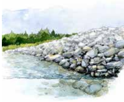
Many fisheries experts believe that the most critical impacts to fish and fish habitat occur, not as a result of a flood event itself, but rather from our response to the flood. Bioengineering is more ecologically beneficial than hard riprap designs—the practice of armouring and stabilizing banks with rock.
