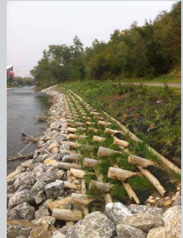
Bioengineering can outperform riprap—the practice of armouring banks with rock.
