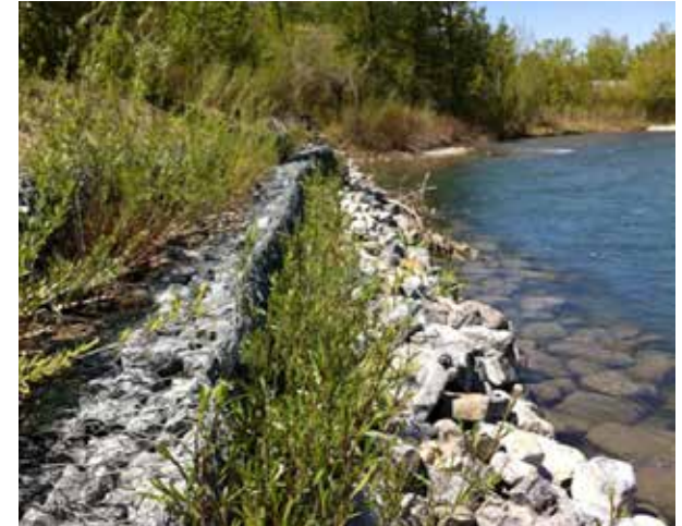
Vegetated gabion project
