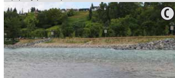
Rip rap and groynes – Sunnyside, Memorial Drive
