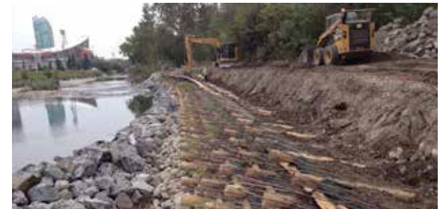
Live timber crib wall across from Stampede grounds during installation, summer 2014
