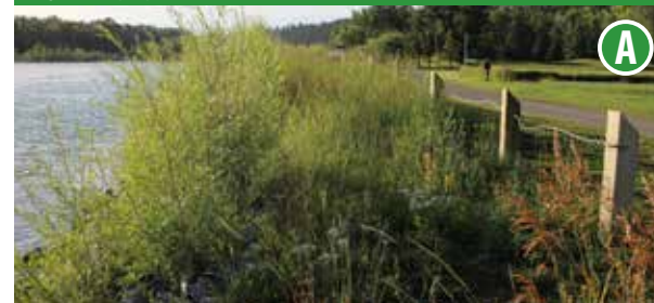
Vegetated rip rap – outfall B134
