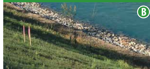
Home Road bank stabilization
