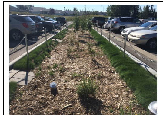
Photo 1-1: Bioretention area, Carburn Park, Calgary, AB
