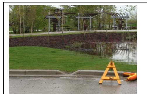
Photo 2-2: Curb cut leading to bioretention area, Walden Development, Calgary, AB
