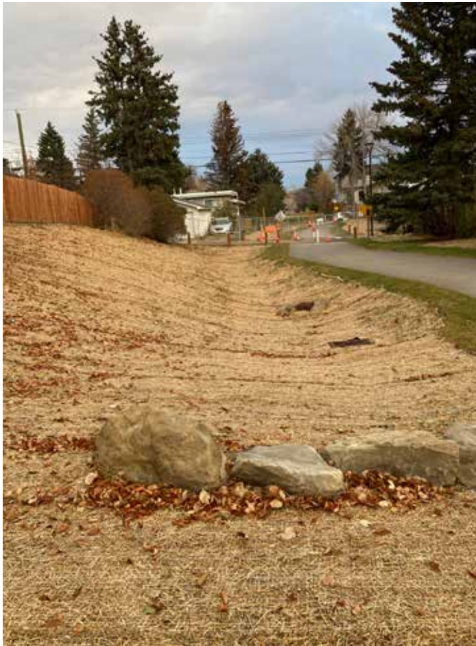
Capitol Hill curb inlet and naturalized swale.
