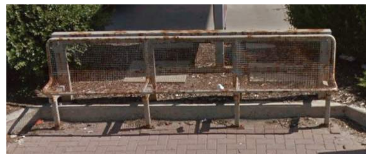
FIGURE 2.11 - EXISTING TRANSIT STOP NEAR 46 STREET NW
