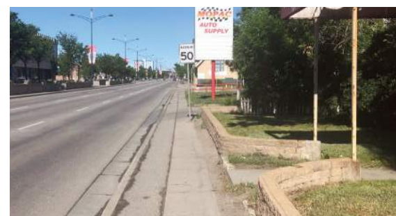
FIGURE 2.13 - TYPICAL SIDEWALK CONDITION ALONG 16 AVENUE NW IN SUMMER MONTHS
