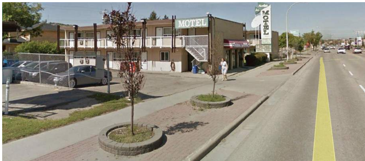
FIGURE 2.8 - TREES IN PITS IN POOR CONDITION BETWEEN MONTEREY AVENUE NW AND 46 STREET NW
