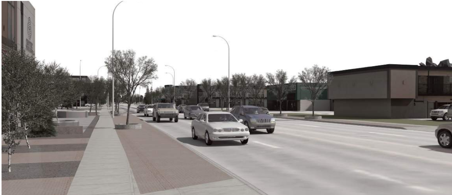
FIGURE 4.09 - TYPICAL EXISTING CONDITION, NORTH SIDE OF 16 AVENUE NW LOOKING EAST BETWEEN 46 STREET NW AND 45 STREET NW
