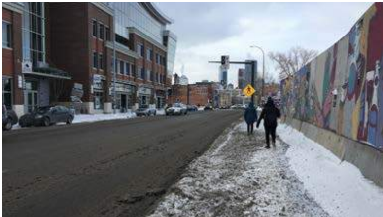
Winter Maintenance Conditions Create Barriers For Pedestrians
