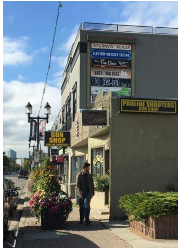
Insufficient Width For Street Furnishings and Pedestrian Circulation
